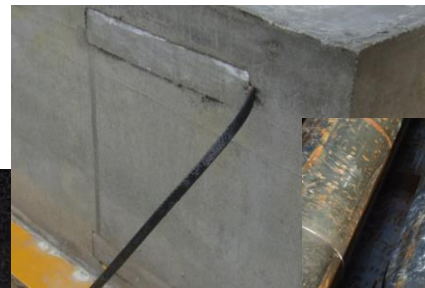
Embedded in concrete structures
